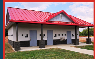
Cedar Stone Park Restroom
